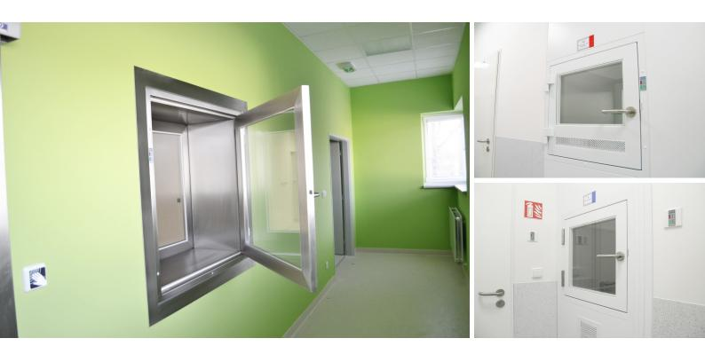
Glazed hinged doors are used in material pass-throughs, which serve to transport material between rooms with different classes of cleanliness.
