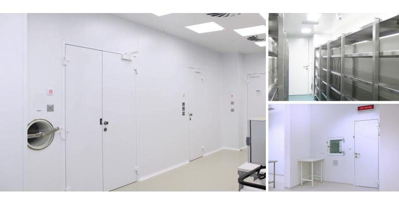
Together with the casing, partition panels and ceiling panels with increased thermal resistance, this door with increased thermal resistance is another component for the construction of cold storage rooms and thermochambers.
