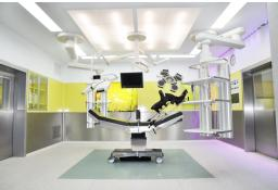
Lamination flow fields are used to create a uniform airflow of specific cleanliness in septic and aseptic operating theatres.
