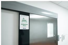
Automatic sliding doors may be adapted to many different access requirements in order to fulfil their function in an optimum and reliable manner. Automatic sliding doors are powered by an AC motor. The motor is controlled by a microprocessor-equipped frequency converter, thus keeping the automatic door under perfect control in every situation, with an emphasis on safety.
