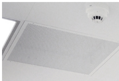
2) Perforated plate with ~30% free area
