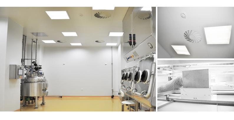
PUROFIL terminal diffusers are intended as an end filtration element in the air distribution system for environments with high demands for the purity of incoming air - such as operating theatres, sterilisation rooms, intensive care units, different areas in pharmaceutical industry, electrical engineering industry, mechanical engineering industry, food industry, etc.
