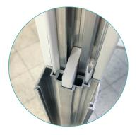
1) Sheath 2) Al frame 3) Al frame 4) Panels with connecting part Mastic
