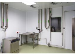
Basic partition panels represent one of the basic elements to construct clean workplaces and areas with maximum safety, sterility, hygiene, easy maintenance and sanitation. Due to the tight connection between the partition panels, spaces created between the panels, the floor and the ceiling are guaranteed to contain overpressure or underpressure in the room, which means that they meet the basic criteria for clean areas, for which these panels were specifically designed and proven.
