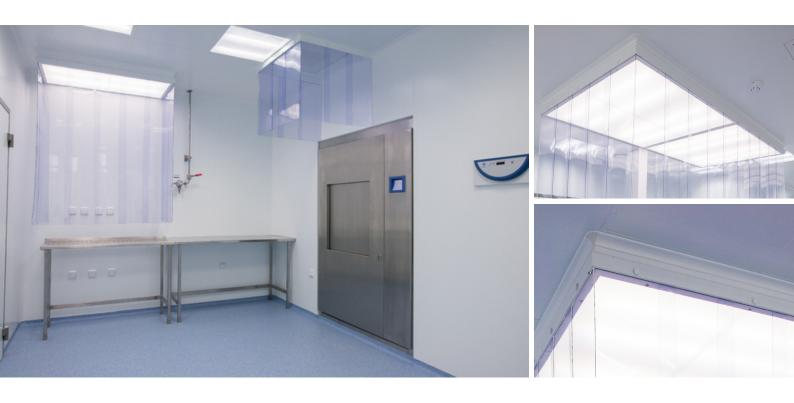
The screens are designed to increase airflow efficiency. They form a closed workplace with uniform airflow under a circulation unit or laminar field.
