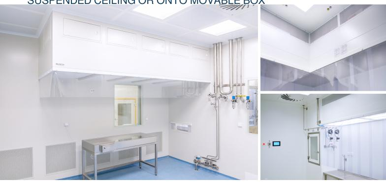
Circulating units are used to supply filtered air to a workplace and to protect the product from ambient contamination.
