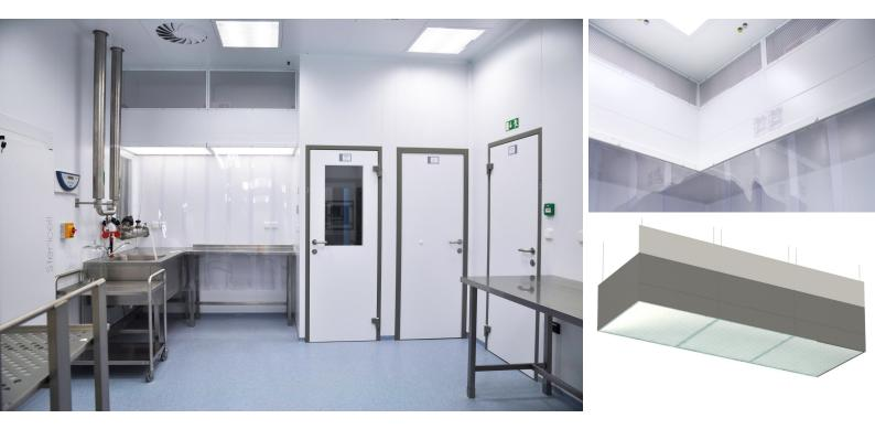
The additional covering of the upper area above the circulating unit is designed with individual metal panels, as specified in Section S3, S4 and combination thereof. The preferred dimensions are 625 and 1250 mm for circulating units 625x1250, 1250x1250.
