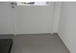
The floor in clean rooms requires high durability and easy cleanability. To ensure the maximum cleanability of the room corners, it is necessary to use covings for a smooth transition between the flooring and the wall. The pre-pressed flooring elements are inserted into the corners to ensure fast and smooth connection. Therefore, PVC-based materials are selected for floors. The particular type of PVC is determined by the designer at the request of the investor.
