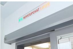
The "DO NOT ENTER" light serves to warn people in a cleanroom of potential dangers associated with entering certain workplaces, such as X-ray radiation or a high-power laser.
