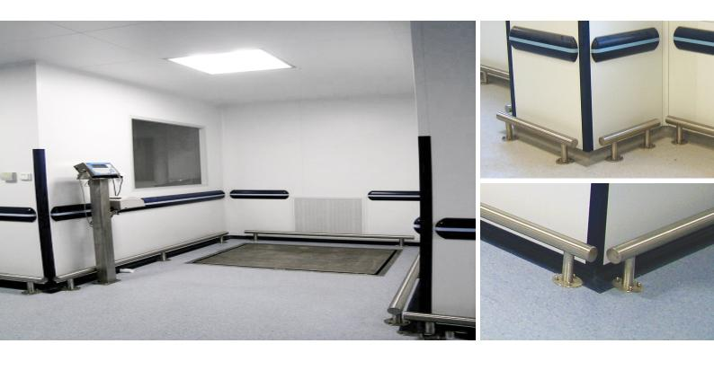
Stainless steel guardrails and corner guards are used to protect partitions from damage during the passage of carts, mobile containers, etc.
