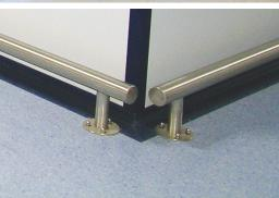
Stainless steel guide rails and corner guards are used to protect partitions from damage caused by carts, mobile boilers etc.
