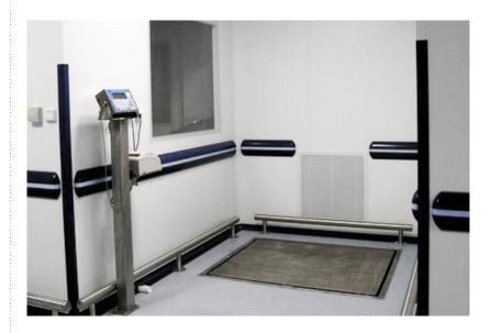
Stainless steel guide rails and corner guards are used to protect partitions from damage caused by carts, mobile boilers etc.
