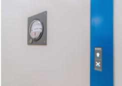
The electronic door signalling system allows cleanroom personnel to follow the prescribed operating regime for the movement of people and material. It consists of two or more signalling boxes located near the cleanroom doors above the suspended ceiling. For door interlocking, electronic signalling supplemented with an electromagnetic lock can be used.
