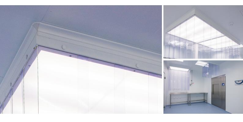
Screens are designed to increase the efficiency of airflow in a clean environment. They prevent the intake of air from the surrounding room and create a closed workspace with a uniform airflow under a circulation unit or laminar field.
