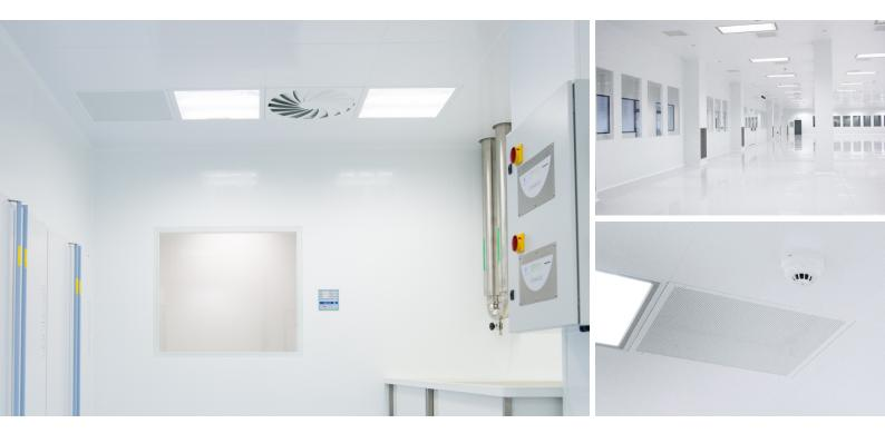
Air conditioning adapters are intended as an end component of the air distribution system.
