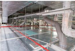
Ceiling panels are designed for the construction of suspended ceilings where limited movement of persons on the top side of the suspended ceiling is expected during installation and service work.
