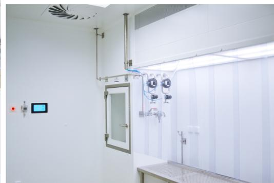
Circulating units are used to supply filtered air to a workplace and to protect the product from ambient contamination. The circulating unit is to be installed in clean rooms of all purity classes. When installing the circulating unit in areas without a defined purity class or in an environment with increased dust generation, a pre-filter is mounted at its suction inlet.
