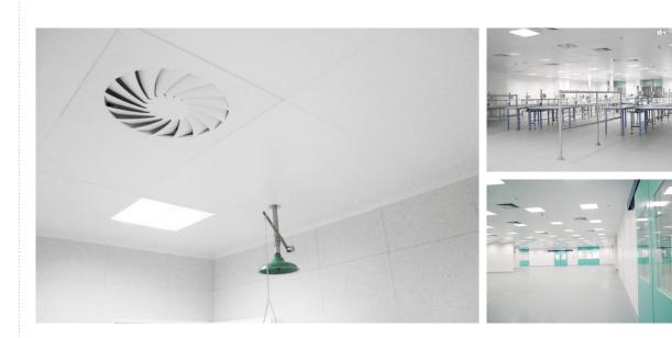
Lightweight metal suspended ceiling is a lowered ceiling structure with a concealed suspension system.
