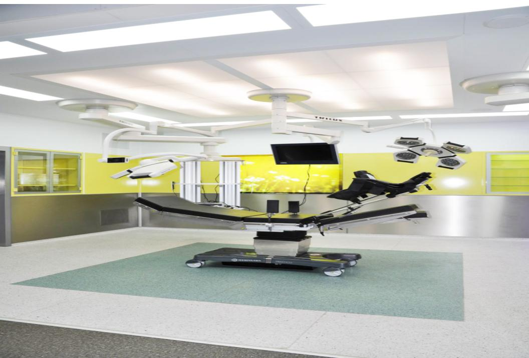
The code is used to specify suspended ceiling panels of atypical dimensions. Ceiling panels of hue RAL 9016 and 9002 are made of painted galvanized steel sheet, thickness 0.6 mm. Panels of other RAL hues are made of galvanized steel sheet, thickness 0.6 mm, surface-finished with thermosetting powder coat, hue according to RAL colour standard.
