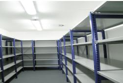
Ceiling panels with increased thermal resistance are used for the construction of cold storage boxes and thermochambers. In these areas, temperature and pressure according to the customer's requirements are maintained. The whole system of connecting panels to each other and to other components (i.e. door casings, ceiling panels, anchoring to the floor) is designed in such a way as to eliminate thermal bridges and minimise heat transfer.
