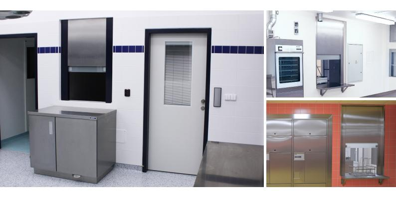
The sliding window is one of the basic components for building clean areas and workplaces with maximum safety, sterility, hygiene, easy maintenance and sanitation.
