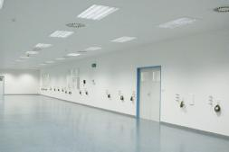
HPL partition panels represent one of the basic elements to construct clean workplaces and areas with maximum safety, sterility, hygiene, easy maintenance, sanitation, and - in particular - chemical resistance.
