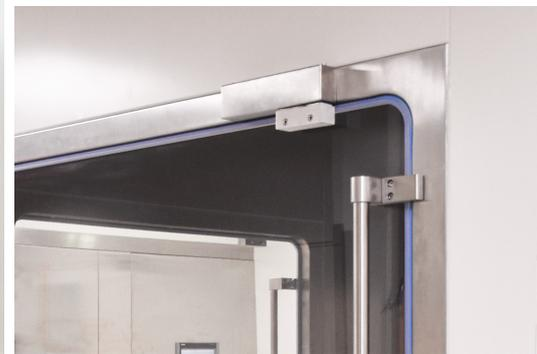
Tight doors together with casing represent one of the basic elements to construct clean workplaces and areas with maximum safety, sterility, hygiene, easy maintenance and sanitation in pressure-independent rooms.
