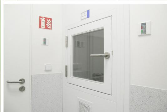
This glazed revolving door is intended for use in clean areas as a material pass-through. It is used to transfer materials between rooms with different classes of cleanliness.
