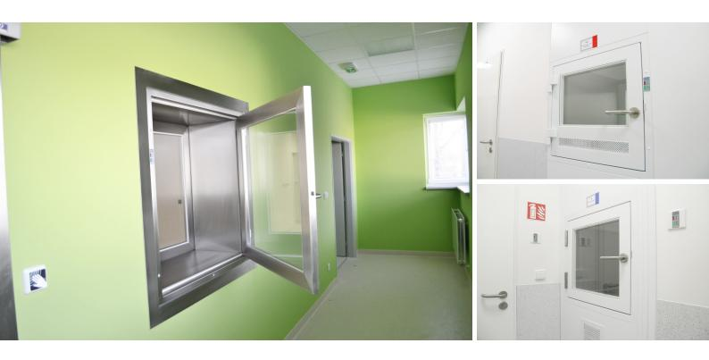
This glazed revolving door is intended for use in clean areas as a material pass-through. It is used to transfer materials between rooms with different classes of cleanliness.
